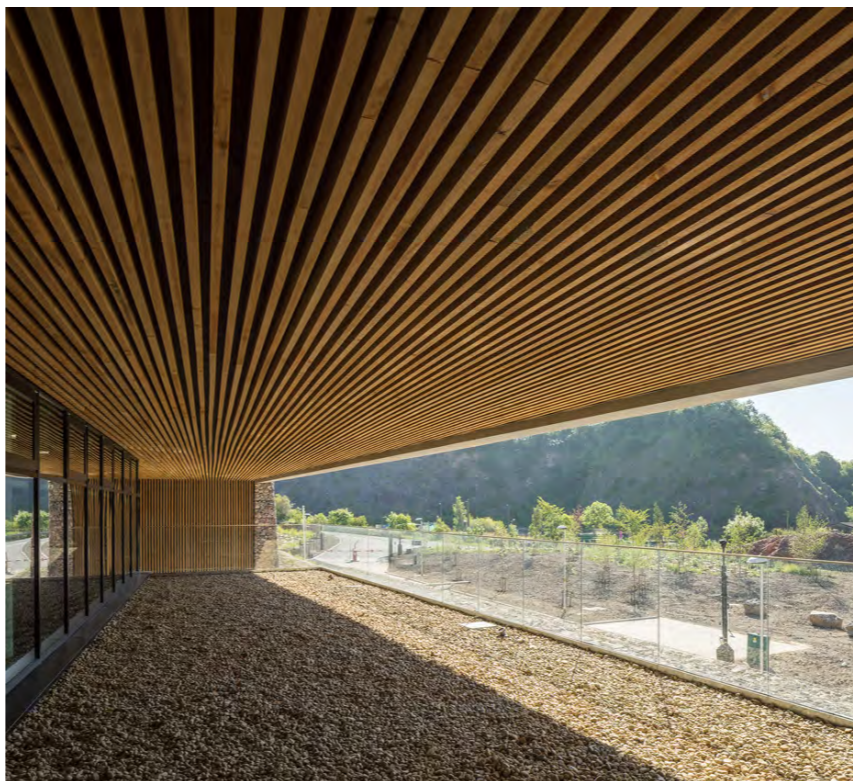
The Blackrock Police Training Centre, Bristol, UK
