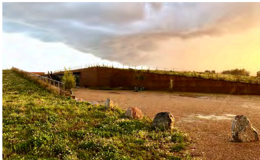
Solrødgård Water Treatment Plant, Hillerød, Denmark
